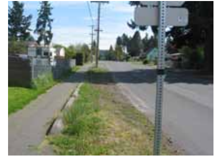
Successful example of SRTS program installing a 'walking path' to improve options for students to walk to school.
