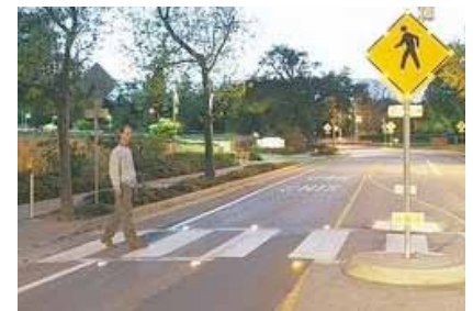
Overhead lighting and/or pedestrian flashing lights in ground or over head will alert drivers when pedestrians are crossing the road.
